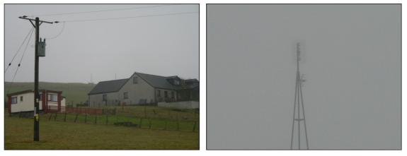
Twatt receives its signal from a self help relay (shown above) which receives the signal from the Weisdale transmitter, boosts it and then redirects it into the valley. The signal from the self help mast was good and is not likely to be affected by the wind turbines. It was also found that there was a very poor signal from the Weisdale mast and a poor signal from Bressay although these were degraded the further down the valley the homes were.
