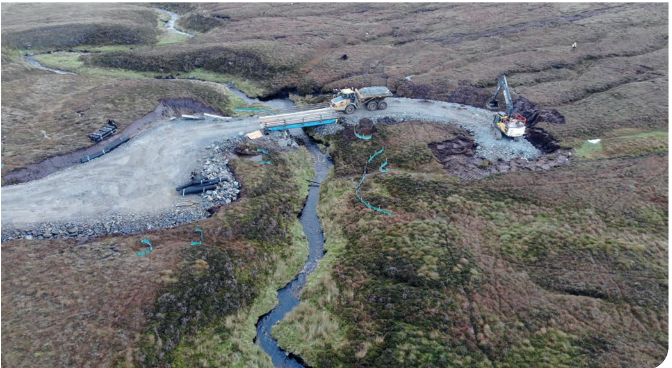
Water crossing over Gossawater Burn.
