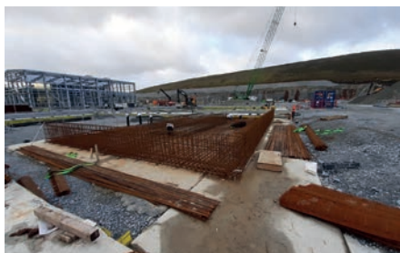
GT1 Bund Steel Fixing.
