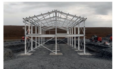
33kV Building Steelwork.
