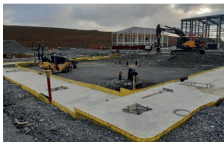
GT2 Strip Found & Duct Install.
