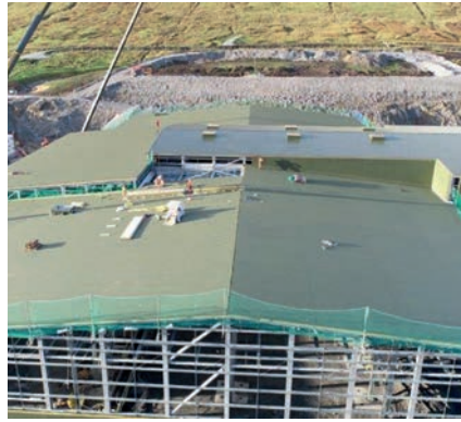
High level cladding HVDC building east.
