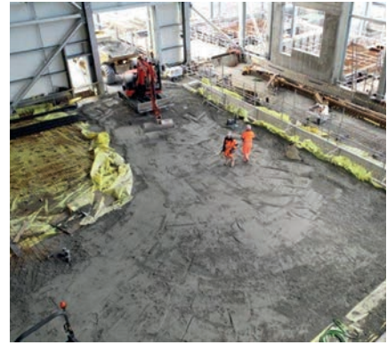
HVDC building floor slab works.
