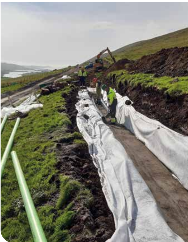
Duct installation works on the hillside parallel to the B9075.
