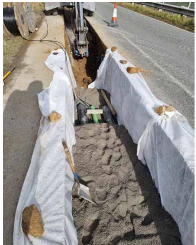
Duct installation works in the A971 carriageway.
