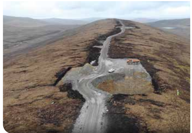
One of the turbine base excavations on Mid Kame.
