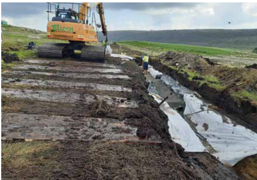
Top soil removal getting underway
