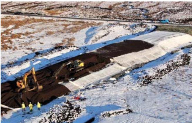
Diggers spreading lightweight Leca.
