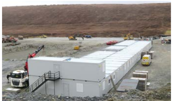
Our site offices are now in place.
