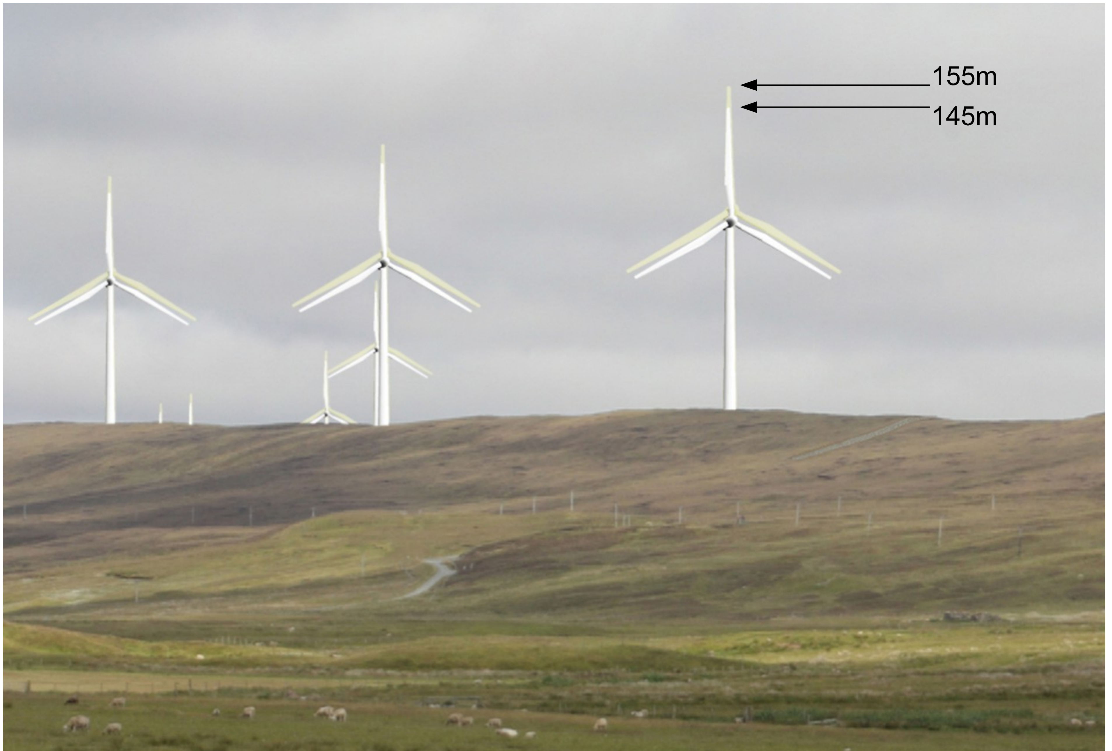
Comparative photograph taken from the Kergord Valley, showing the proposed difference between the consented 145m tip height and the proposed 155m maximum tip height. More detailed comparative visualisations will be available in the application.
