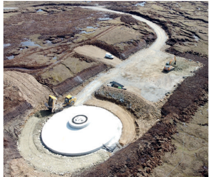
Backfill foundation with selected graded stone up to top of concrete.
