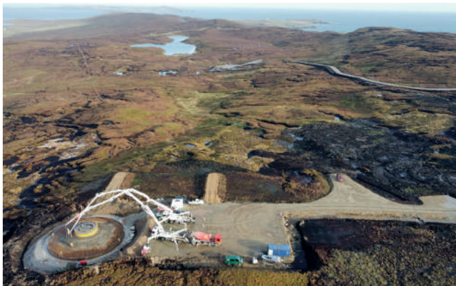
Turbine foundation shuttered and concrete poured.
