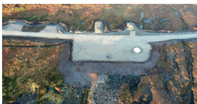
Construct "blade fingers" and two auxiliary hardstands.
