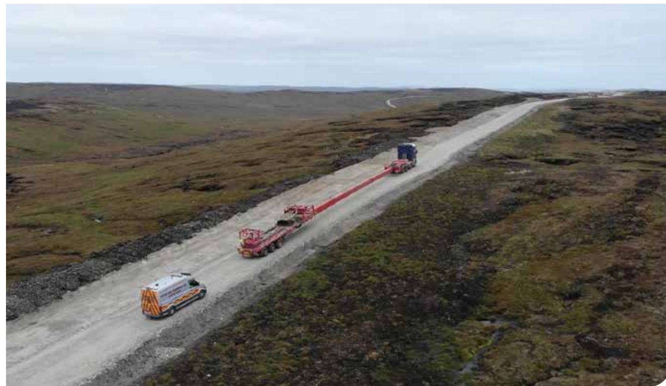
VEWF's turbine supplier, Vestas, recently supervised a "dry-run" on site ahead of turbine component deliveries beginning in January next year. This photo shows one of the specialised trailers, which will deliver turbine blades, heading into the east of the site.
