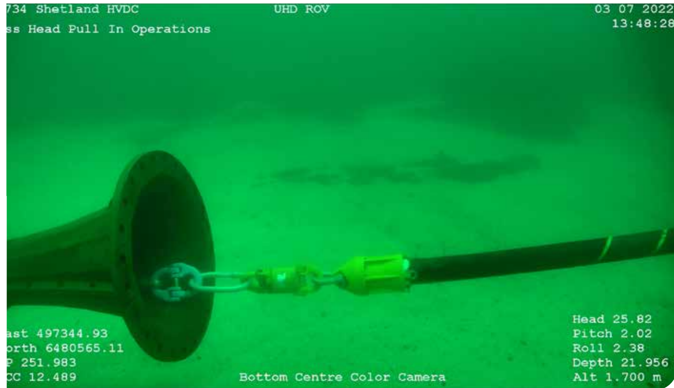
Cable pull-in rigging entering the bellmouth.
