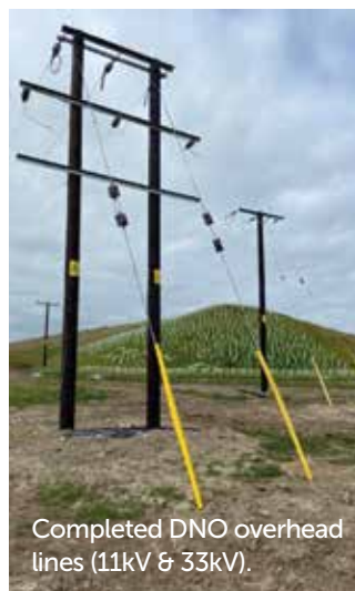
HV equipment completed in Blackhillock Bay.
