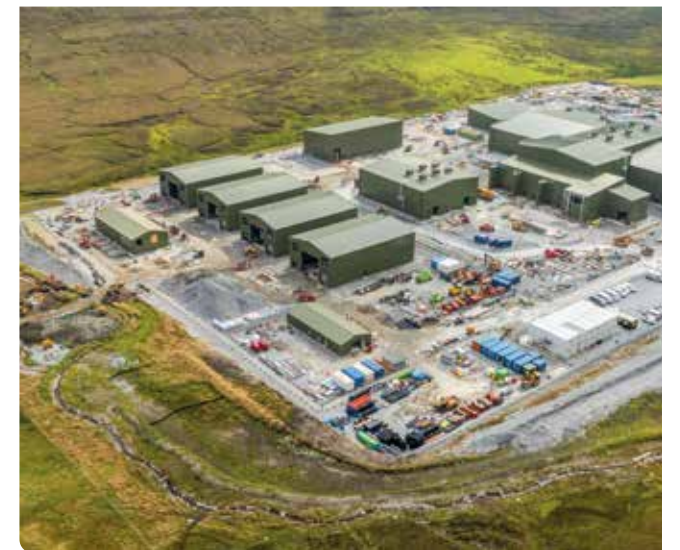
VEWF Substation is located on the left of this picture.
