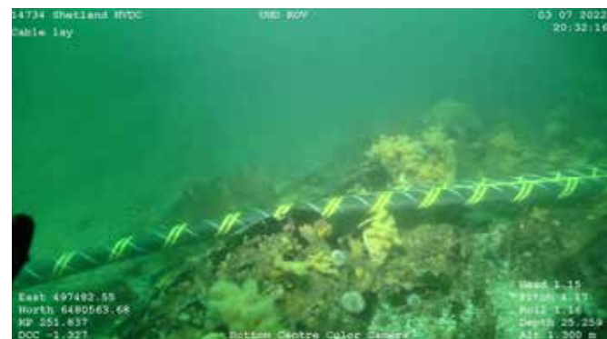
Example of cable lay.
