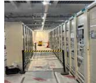
GIS Hall – Being Prepared for Gas Insulated Switchgear (GIS) Installation.
