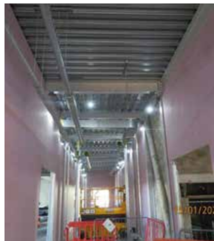
Internal partition walls in control building.
