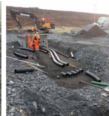
Ducting being laid to connect to troughs.
