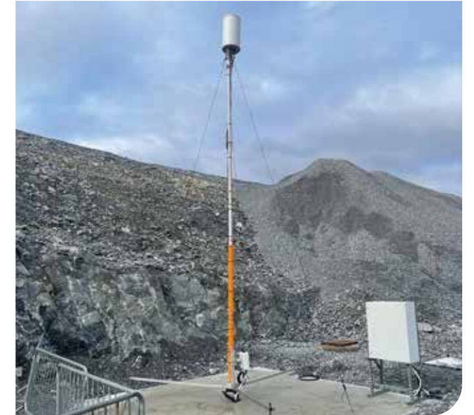
5G Mast installed at Kergord.
