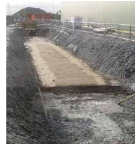
Preparations for trough bases.
