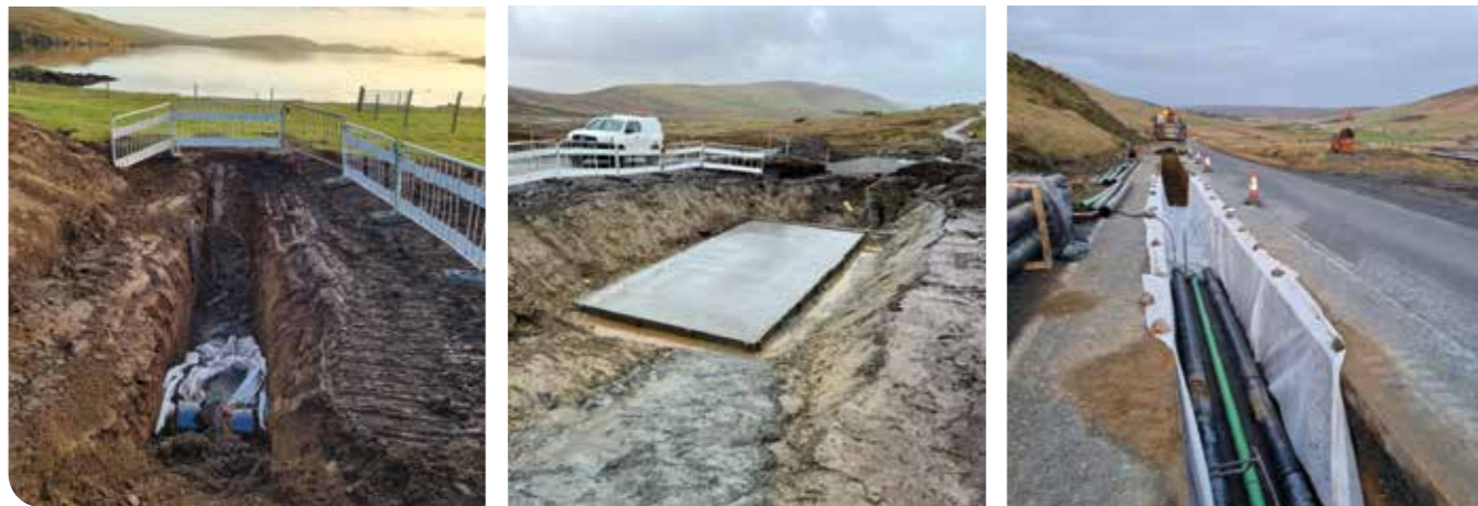
Joint bay Duct Installation works A971.
