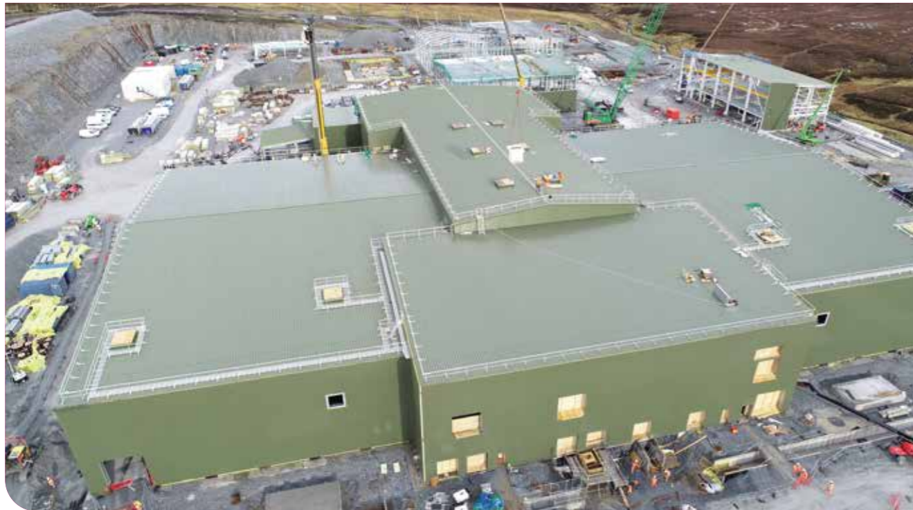
Aerial View – January 2022.
