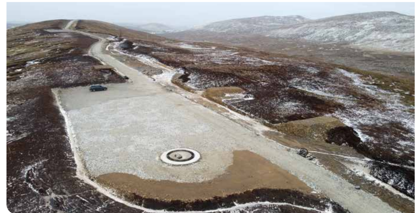
A backfilled turbine base with crane hardstanding on Mid Kame ready for cabling work and final verge reinstatement to commence. The wider area around this base is one of the designated peat restoration areas within VEWF's approved Habitat Management Plan.
