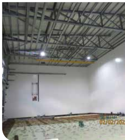
Fireproof internal cladding.
