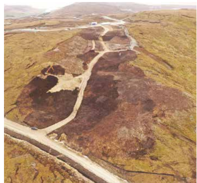
Borrow pit KBP02, West of Kergord. Layers of peat are being applied to exposed rock seams, ahead of final reinstatement.
