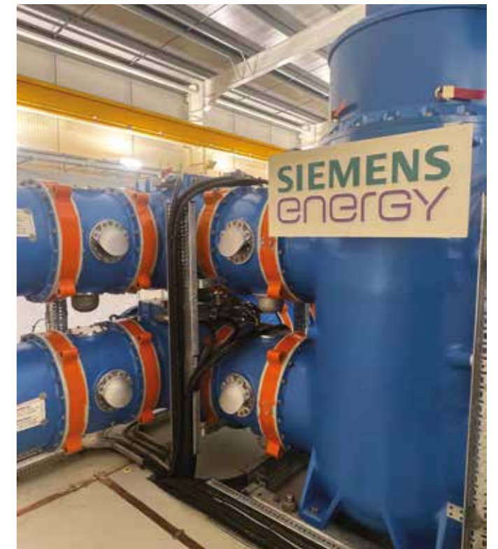
Painting gas tight barriers
