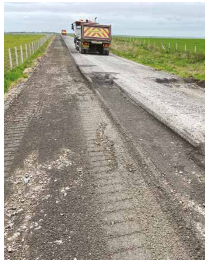
Haul road being removed
