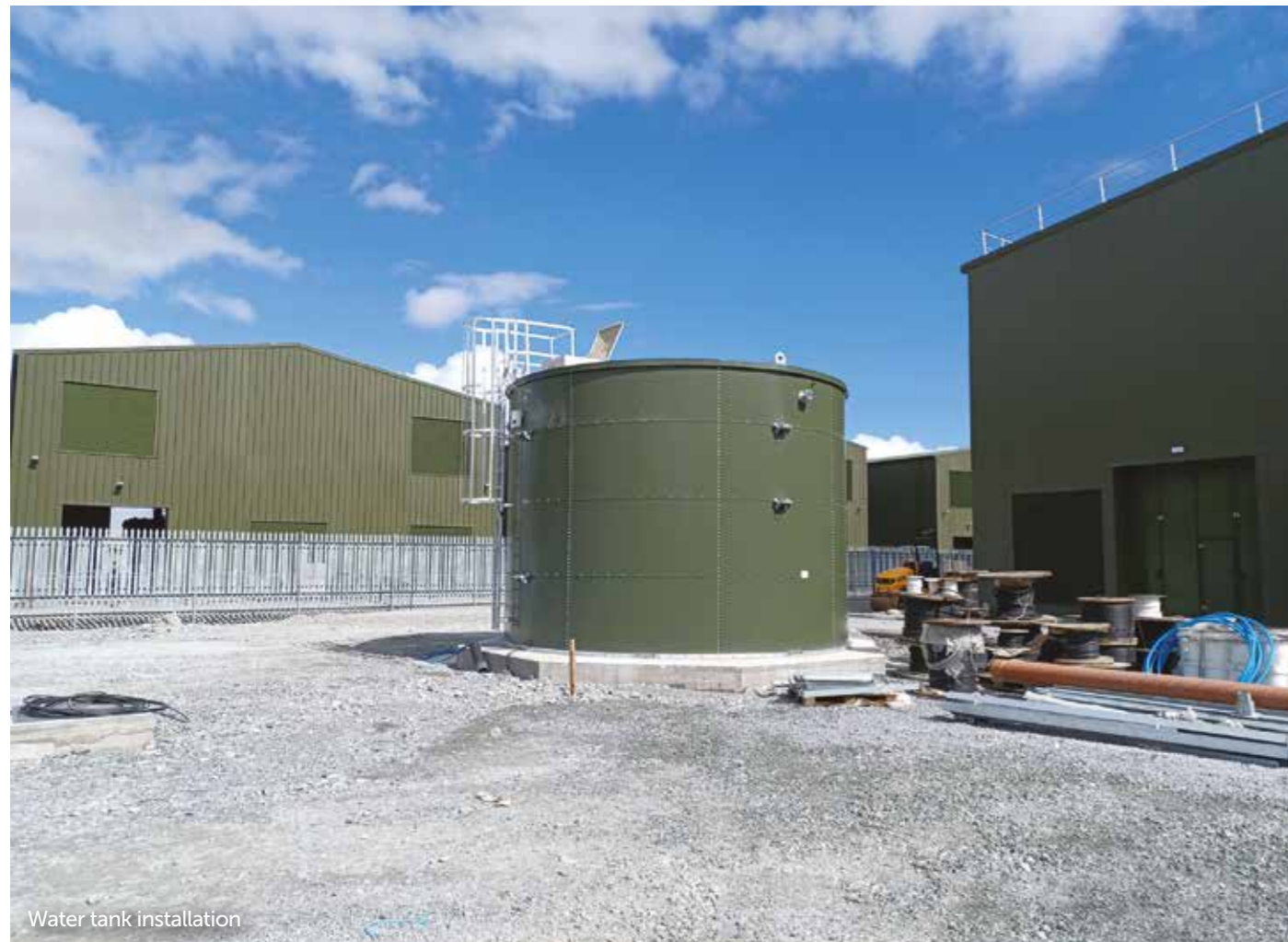
Landscaping works ongoing and water tank installation
